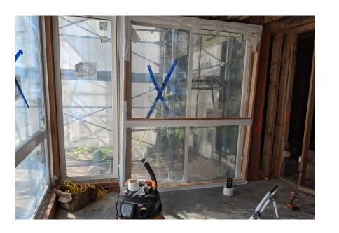
ASTM E783 applies to both residential and commercial buildings with exterior windows, doors, or curtain walls. However, it is more commonly used in commercial buildings and large multi-unit residential projects, where stricter energy efficiency and airtightness standards are required. In this test, a custom chamber is built and attached to a window. Then, a vacuum is pulled on the chamber to test for air leakage.
